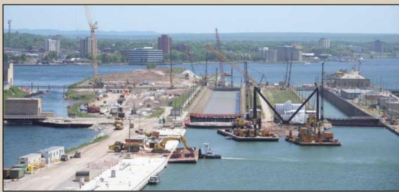
CONSTRUCTION THIS YEAR on the new lock at Sault Ste. Marie includes placement of new steel sheets, concrete cap placements on the upstream approach walls, marine excavation in the upstream and downstream channel, cofferdam construction preparation, abatement of hazardous materials and demolition of existing structures. The trades will also be undertaking construction of a new bridge to the hydro power plant. Photo credits: U.S. Army Corps of Engineers
