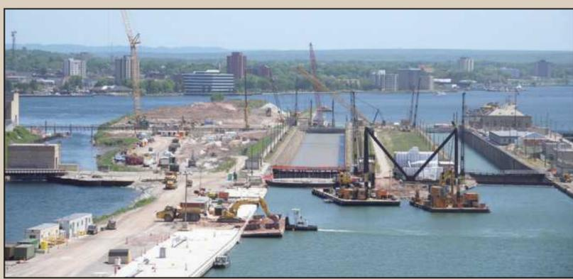
CONSTRUCTION THIS YEAR on the new lock at Sault Ste. Marie includes placement of new steel sheets, concrete cap placements on the upstream approach walls, marine excavation in the upstream and downstream channel, cofferdam construction preparation, abatement of hazardous materials and demolition of existing structures. The trades will also be undertaking construction of a new bridge to the hydro power plant. Photo credits: U.S. Army Corps of Engineers
